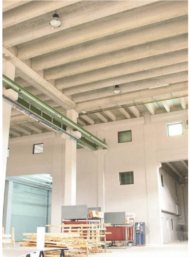
Industrial building with TT slab on top
