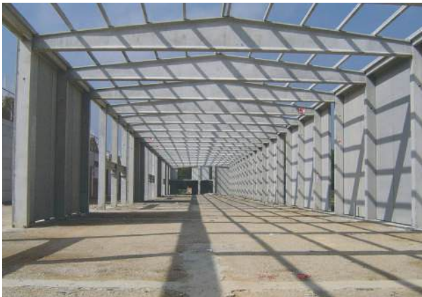
Industrial building with roof beams installed over Delta beam
