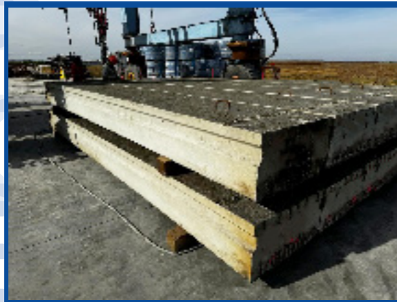
T-shaped precast concrete elements for roads and bridges (L0, L1, 2, L3) Up to 2 pieces per day.
